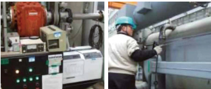
1st leak test
